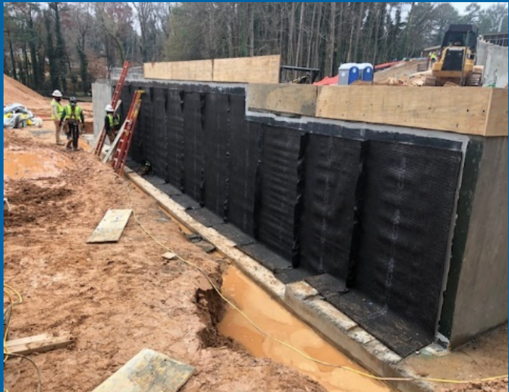
Drainage Mat Installed at Foundation Wall
