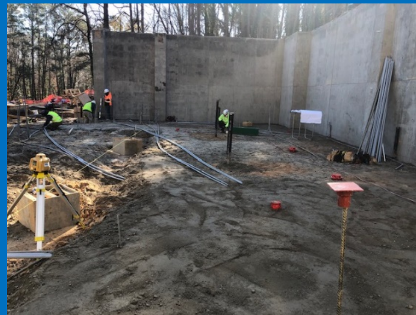
Electrical UG and Slab Prep at Gymnasium
