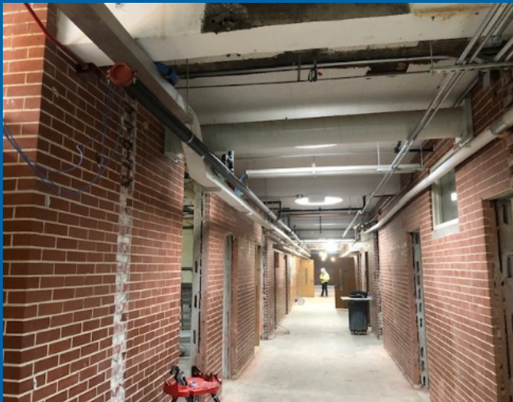
SW Wing Fire Protection Complete and Tested
