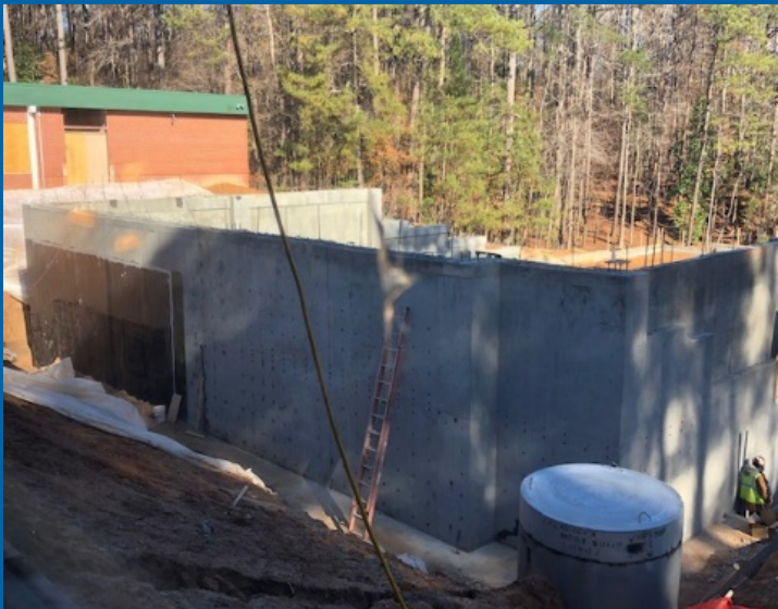
Forms Removed from Concrete Pour
